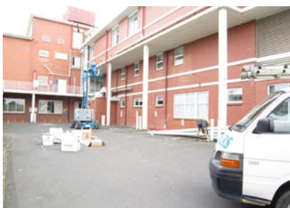
Diverting rainwater downpipes to the storage tanks.
