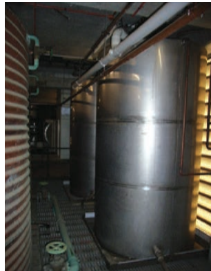
Recycled water header tanks
