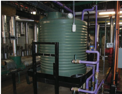
Steriliser water collection tank
