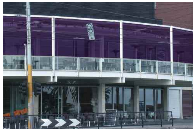
Figure 2. Smoking would not be permitted on the balcony. Note: the shaded area depicts a drawn awning.
