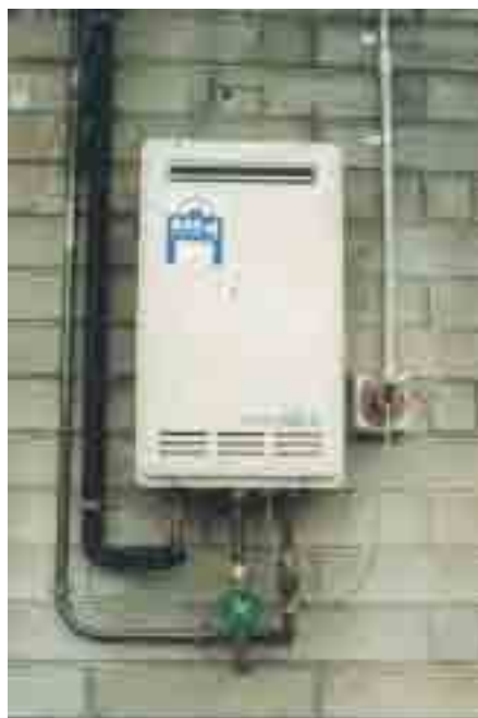
Figure 5 Instantaneous hot water system
