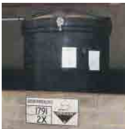
Figure 3 Hazchem signage for bulk dangerous goods
