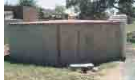
Figure 4 Backwash tank
