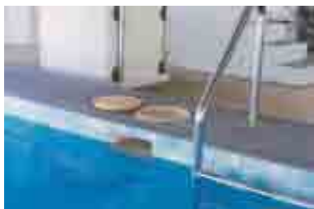
Figure 27 Skimmer box and lint trap
