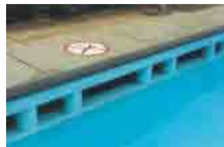
Figure 26 Overflow channel on an older outdoor pool
