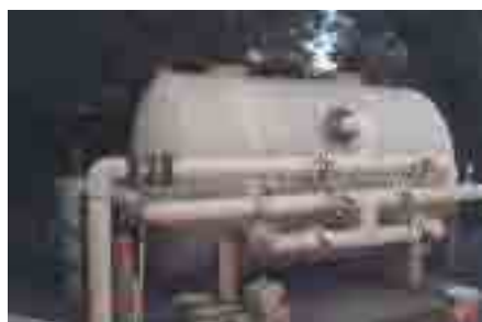
Figure 29 Medium rate pressure filter for larger pool
