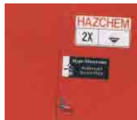
Figure 2 Hazchem signage for packaged dangerous goods
