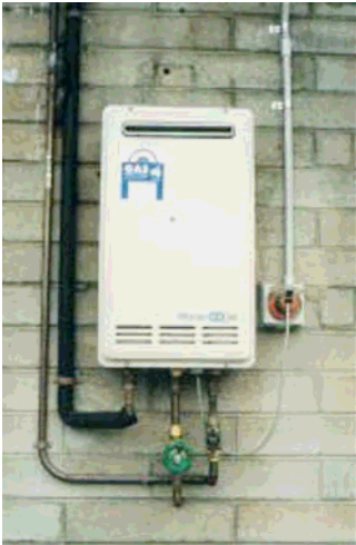
Figure 6 Instantaneous hot water systems
