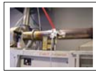
Figure 2(c) Extraction Fan
