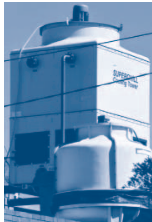
Two common types of cooling tower
