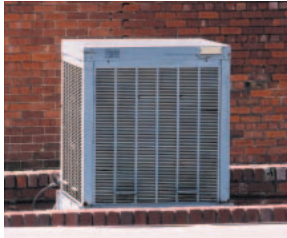
Evaporative Cooler: These units have not been linked to cases of Legionnaires' disease
