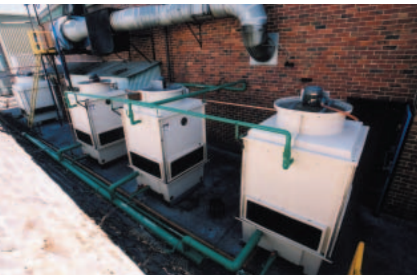
Cooling tower system: A series of inter-connected cooling towers that form part of a cooling tower system
